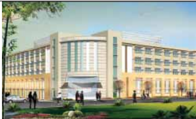
The new Software Development Block at Mysore DC
