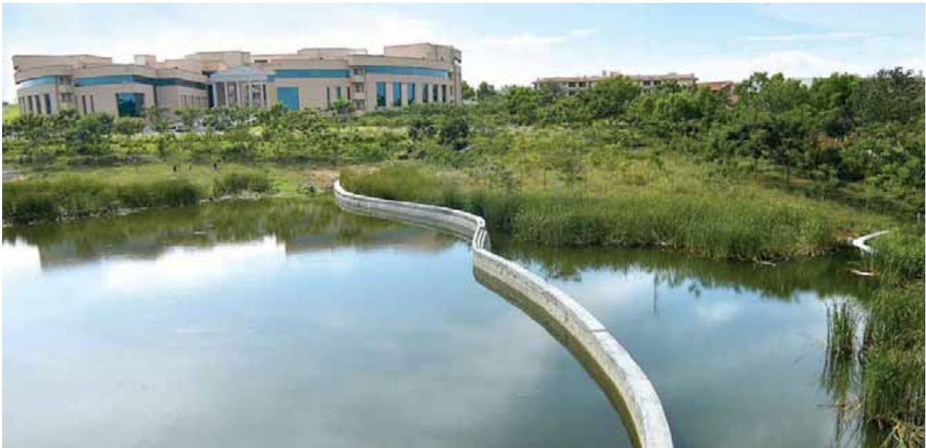
Rainwater harvesting area in our Mysore campus
