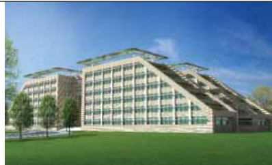
The new Software Development Block under construction at Hyderabad DC
