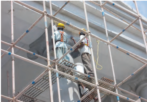
Construction in progress at our Mysore campus
