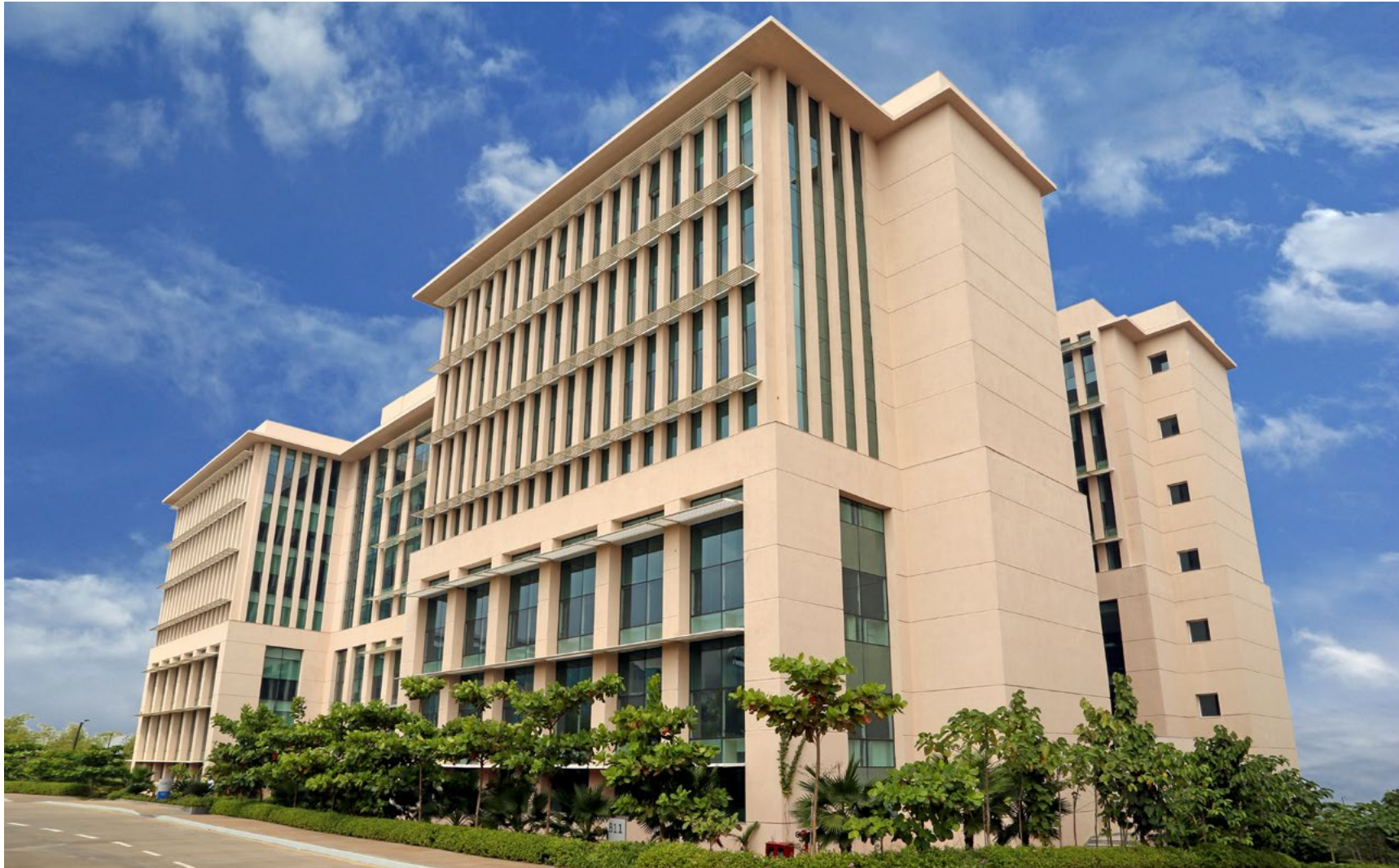
Infosys SDB 3, Mangaluru : The building design demonstrates nearly 33% reduction in energy consumption compared to ASHRAE baseline standards. With the implementation of efficient water flow and flush fixtures like aerators, waterless urinals, flow restrictors etc., water wastage has been minimized extensively.
