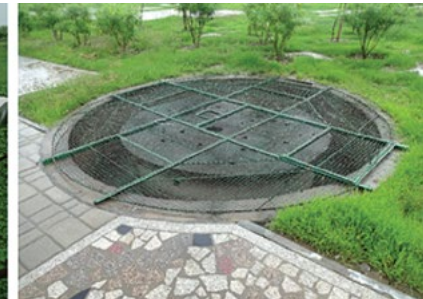
Groundwater recharge well at Jaipur Campus
