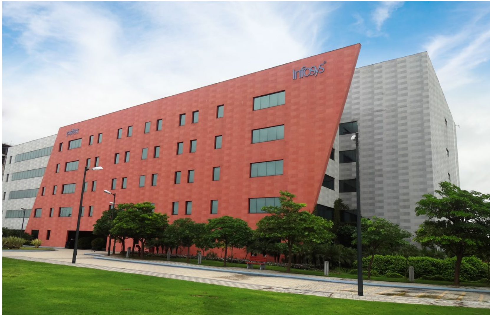
Infosys BPO 1, Jaipur: This building demonstrates nearly 33% reduction in energy consumption as compared to the ASHRAE baseline standards, and uses four modes of cooling systems – direct evaporative cooling mode, indirect evaporative cooling mode, free cooling mode, and chiller mode.
