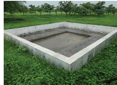
Rooftop rainwater harvesting tank at Jaipur Campus
