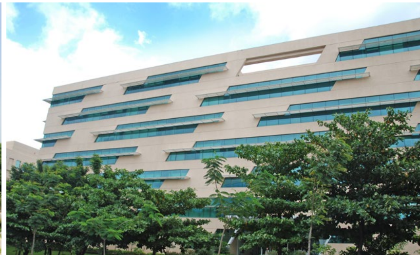
Infosys BPO 2, Pune: The building design demonstrates about 47% reduction in energy consumption compared to ASHRAE baseline standards and uses efficient Chilled Beams system for cooling instead of conventional air conditioning.
