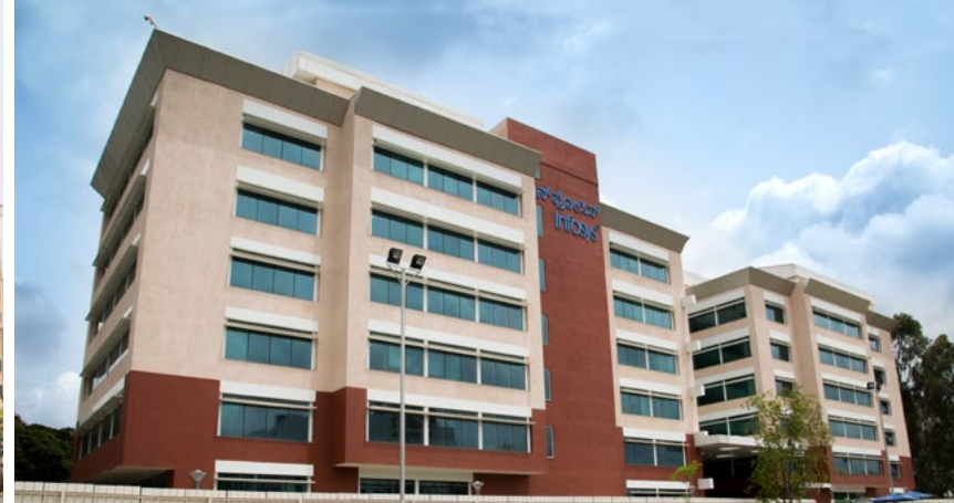
Infosys M&C Building, Bengaluru: The building design demonstrates nearly 42% reduction in energy consumption compared to ASHRAE baseline standards and is the first building in India to implement radiant panel-based cooling system.
