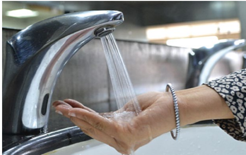
Water faucets with pressure compensating aerators
