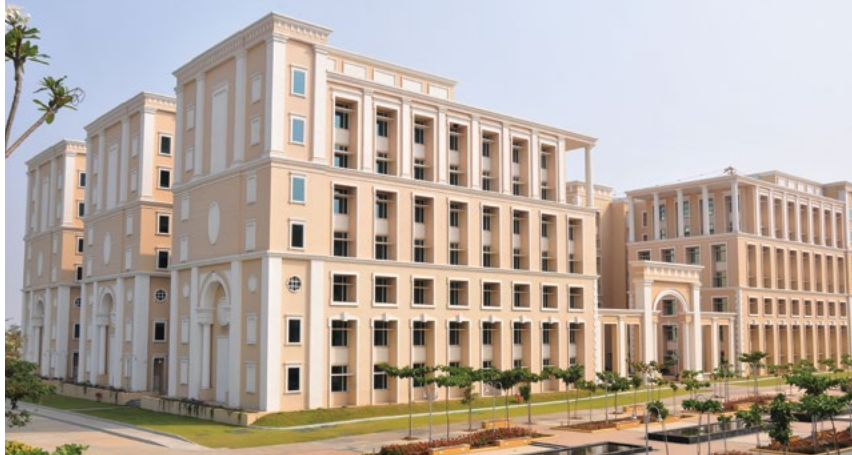
Infosys SDB 6, Mysuru: The building design demonstrates nearly 39% reduction in energy consumption compared to ASHRAE baseline standards. Nearly 78% of the office space is naturally lit and does not require lights during the day and about 93% of occupied spaces have access to outside views.
