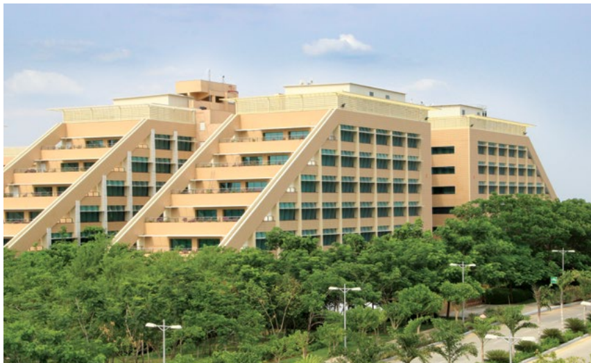
Infosys SDB 1, Hyderabad: This building is the first radiant cooled commercial building in India and the biggest comparison of HVAC system in the world. Daylight and vision panels ensure over 91% of occupied spaces have natural light and all employees have access to views, adding to comfort and productivity.
